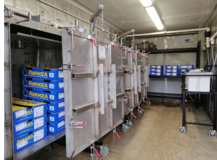
PH 3 treatment facility (500-L chambers)
